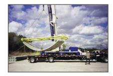
A rope is attached to each end of the spreader so when it is lifted, personnel can guide the mat onto the truck. This insures an evenly distributed load for transportation to the job site.
