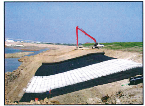
Geotextile and mats being installed
