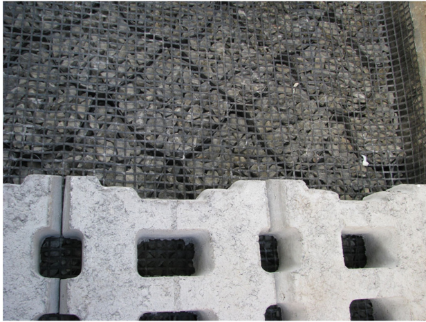
Figure 2 – EPEC System During Flume Installation
