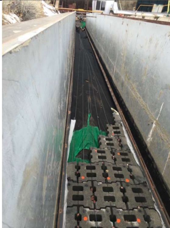
Figure 3 – Flume Post Failure Hydraulic Jump Test ID 2
