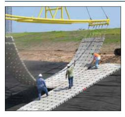
SHOREBLOCK® BD mattresses are pre-assembled to the size specified for the project. Fabrication of a SHOREBLOCK® BD mat is accomplished by threading polyester cable in both directions through a series of
